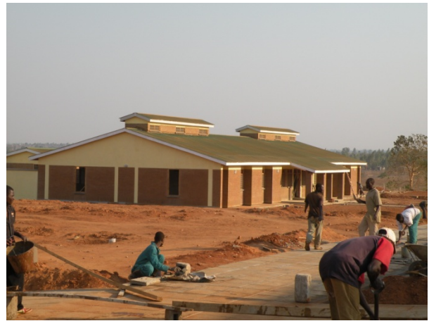
Preparing grounds around Girls' Hostel at LJSS
