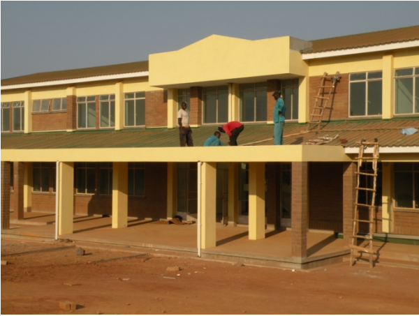
Putting some final touches on entrance to Administration Block of LJSS!
